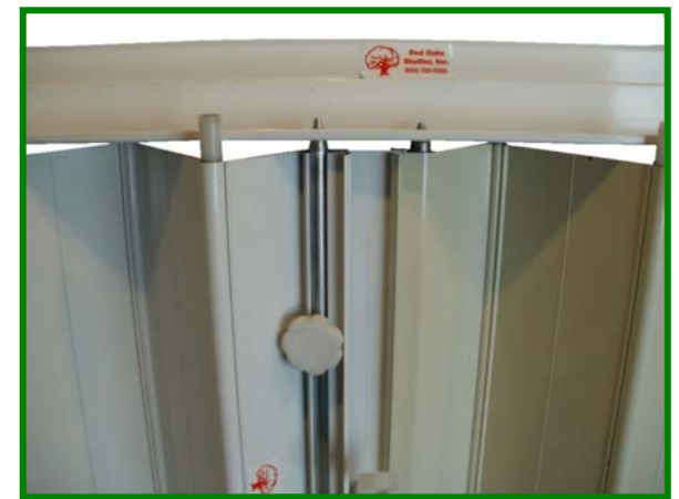
HV Accordion Shutter locking rod close up
